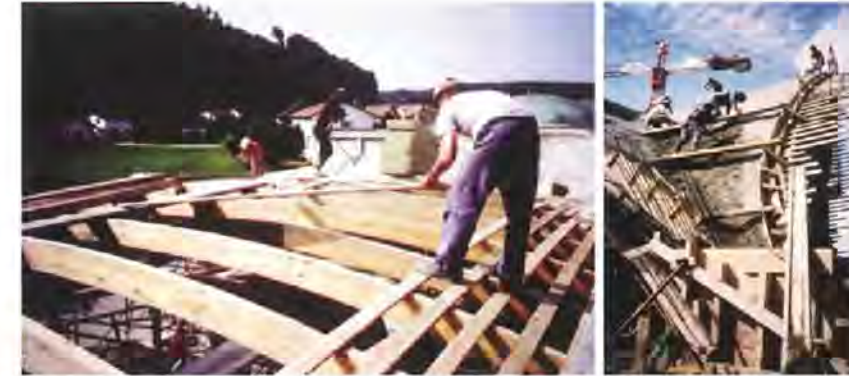
Timber formwork construction and casting of Isler shells (taken from Bösiger, 2011)
