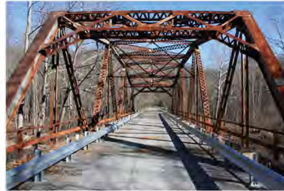
Dunlap's Creek Bridge
